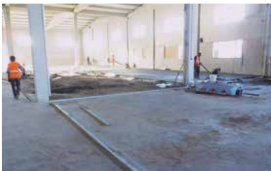
Laying the concrete floor before the panels are fitted
