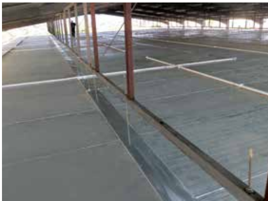
Ceiling suspender and joints used to connect the ceiling panels
